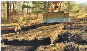
REMOVING THE BRIDGE
