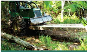
INSTALL BRIDGE PANELS
