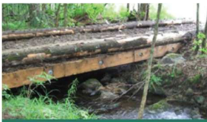
INSTALL BUMPER LOGS
