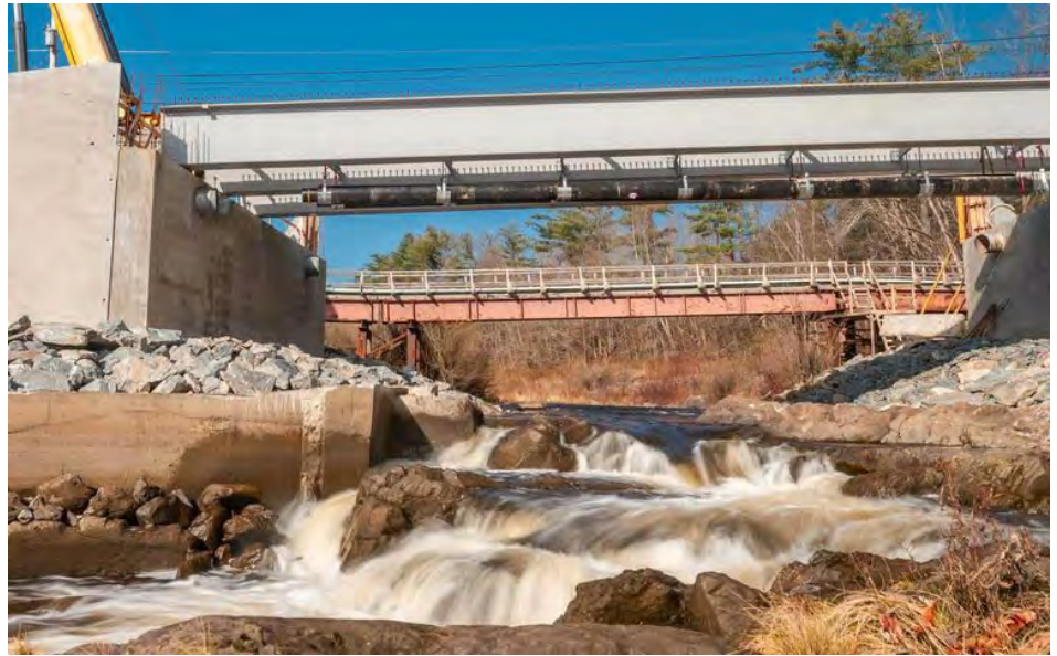
The Grist Mill Bridge Over Souadabscook Stream
