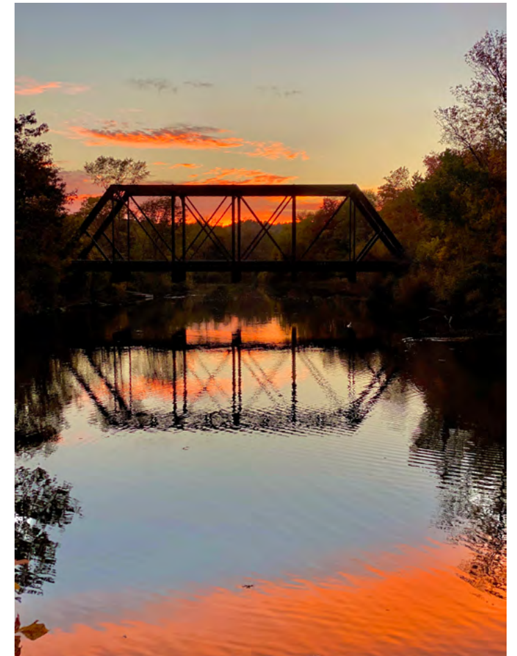
Trestle Bridge over the Royal River Photo: Karin Ornstein
