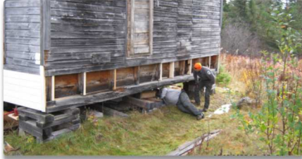
Checking Sill Jay Young and Tyler Stockwell inspect the project.
