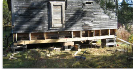
Sill Replaced That's a 24 foot 8"x 8", not easy to find.
