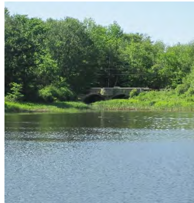
B – Pond with inlet stream on far side
