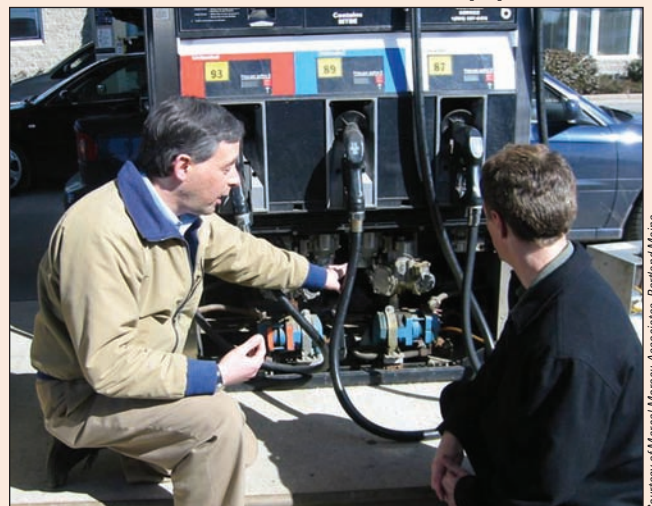
Courtesy of Marcel Moreau Associates, Portland Maine.
