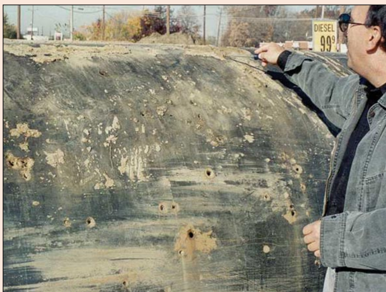
Courtesy of Marcel Moreau Associates, Portland Maine.
