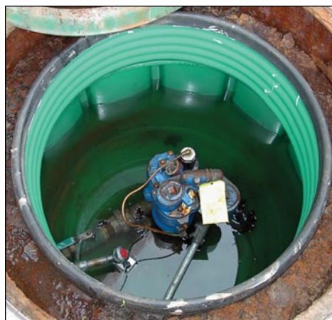
An automatic tank gauge in alarm.
