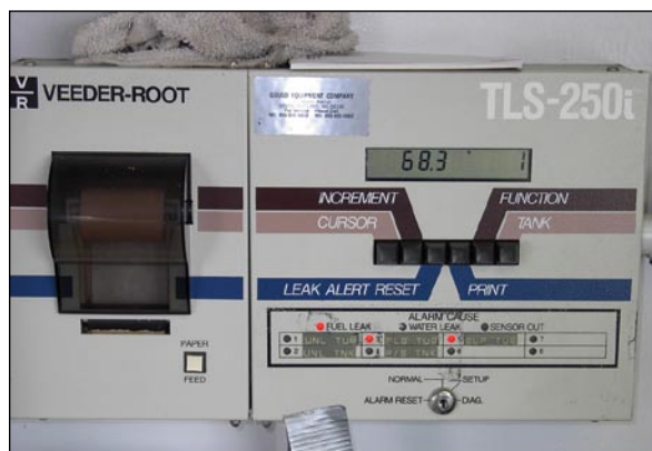
An automatic tank gauge in alarm.
