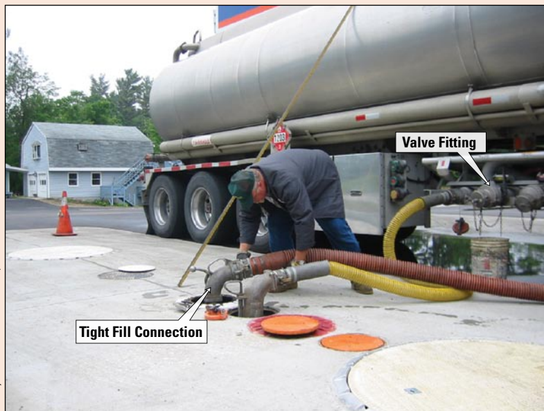
Courtesy of Marcel Moreau Associates, Portland, Maine.
