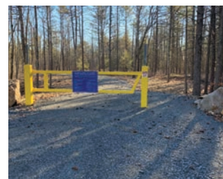
The gate is complete, painted and the rules of use sign and gate number attached.
