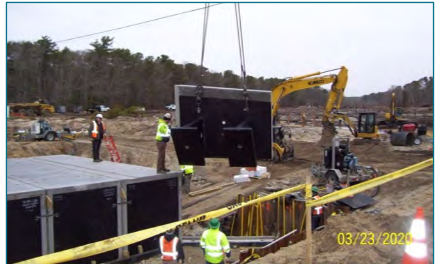
FIGURE B.11 - A pre-cast wingwall installation for a three-sided rigid frame with pre-cast footings. Coonamessett River, Falmouth, MA. Image source: Chris Bennett.
