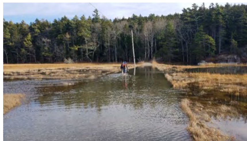
FIGURE B.3 - Example of a "fair-weather" road that overtops with a similar frequency as the adjacent marsh in Phippsburg. Photo by Erno Bonebakker.
