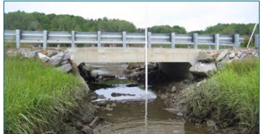
FIGURE B.7 - A three-sided concrete rigid frame structure, installed on Wallace Shore Road (private) in Harpswell, ME. Image source: Matt Craig.
