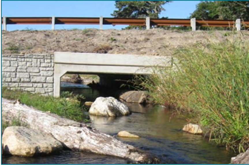
FIGURE B.4 - A reinforced concrete box structure with prefabricated wingwalls and an installed channel bed. Structure size in this example was five feet rise by ten feet span. Eel River, Plymouth, MA. Image source: Inter-Fluve.
