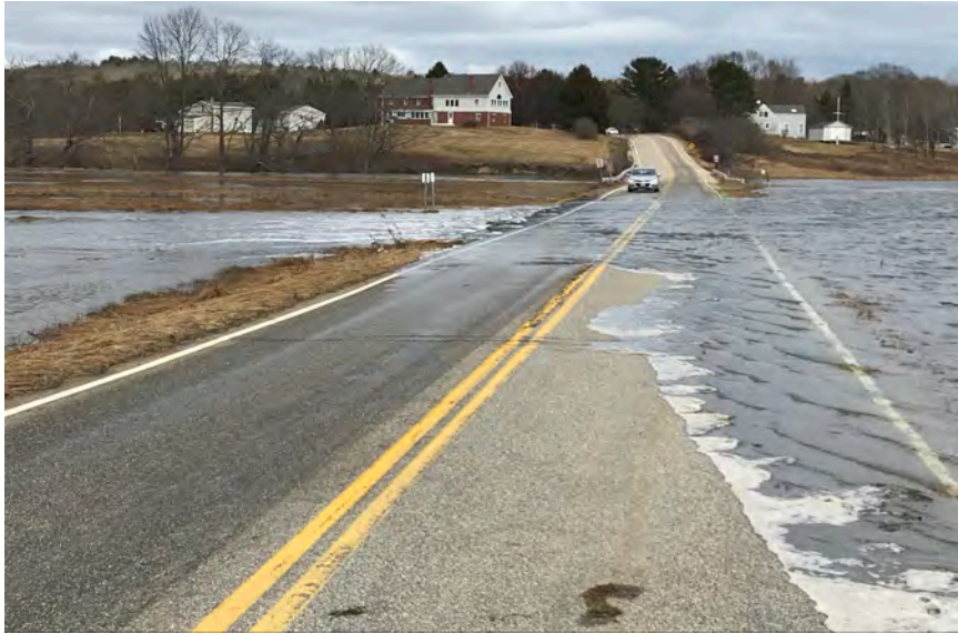
FIGURE 1.11 - Roads flooded by tidal waters can block evacuation routes, cause slower response times by emergency medical services, and impair access to important services. Photo source: Town of Cape Elizabeth.
