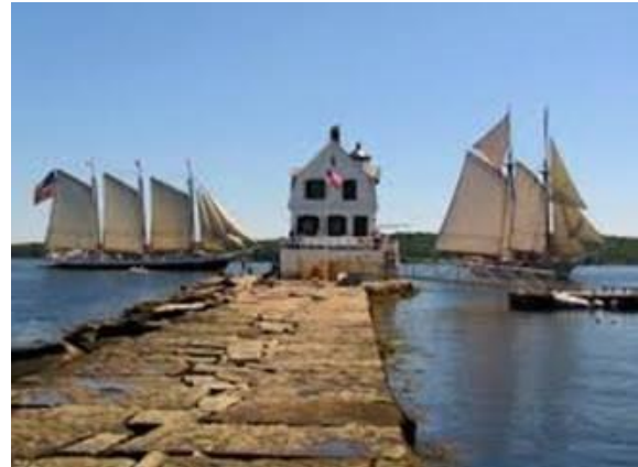
Rockland Breakwater Lighthouse
