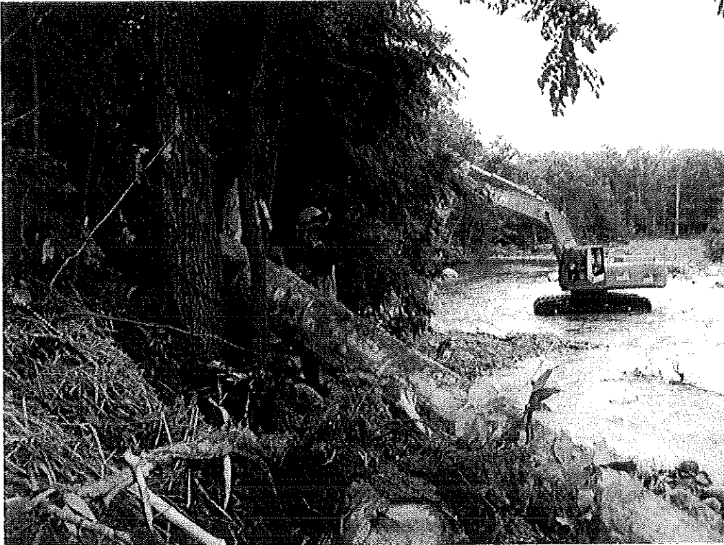
Bar buddies being placed between rock vanes in Sunday River, 2008, to stabilize shoreline.
