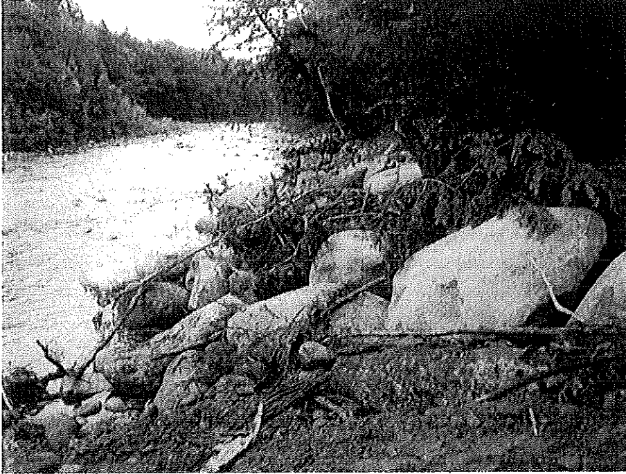
Rock vanes, Sunday River, installed 2008 to divert flow away from bank, trap sediment, narrow stream, and create pools.
