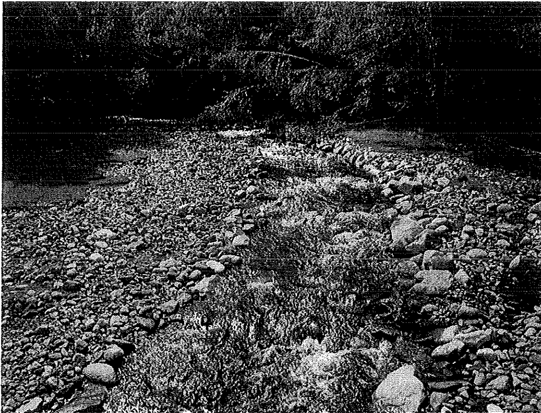
Keystone rock structures, South Bog Stream, four years after construction, showing concentrated flow and riffle-pool sequence.
