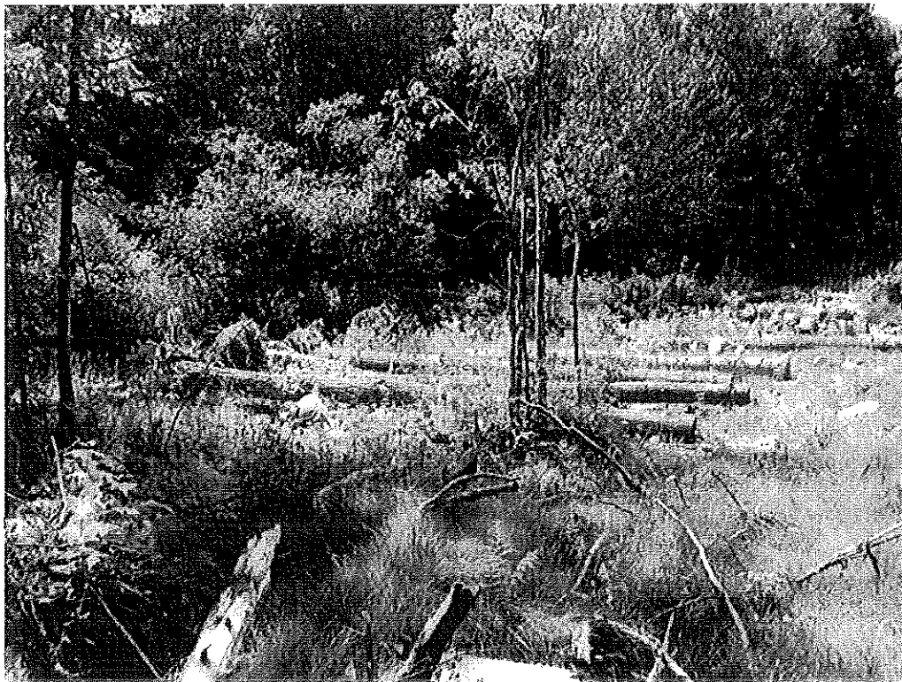
Root wads, South Bog Stream, placed to trap sediment and narrow an overwidened reach.
