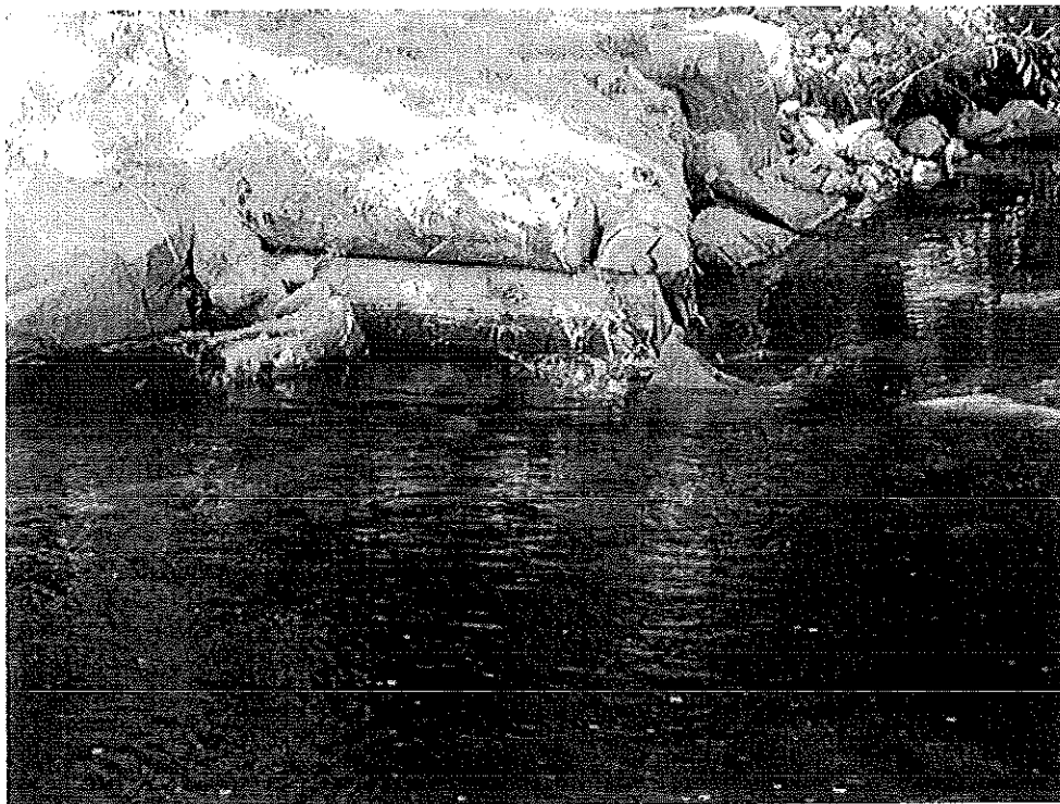
Log wing deflector, South Bog Stream, installed 2004 to narrow channel and trap sediment.
