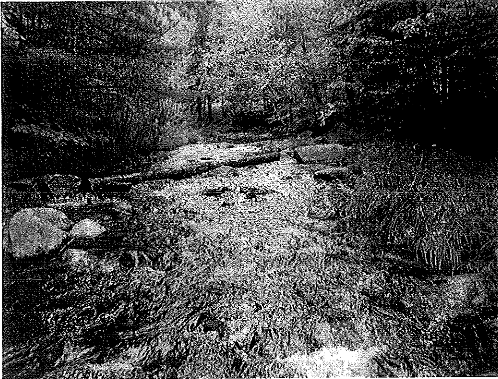
Cabled log, Sandy River, placed in 2007 to divert flow and narrow channel.
